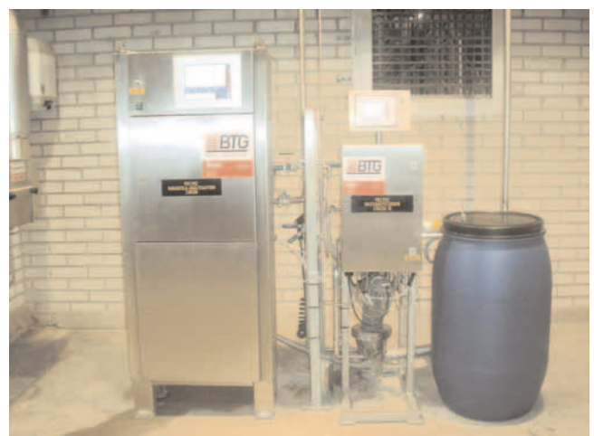
Figure 3 - Installation at PM level
